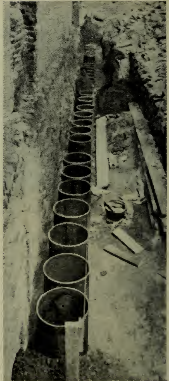
FIG. 4. PLACING FIRST THREE-FOOT LENGTHS OF CASING UNDER WALLS.
